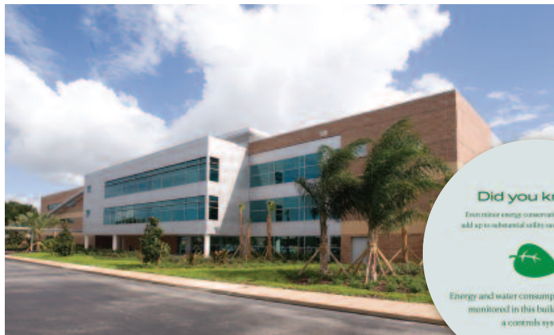
Allied Health and Sciences Building
